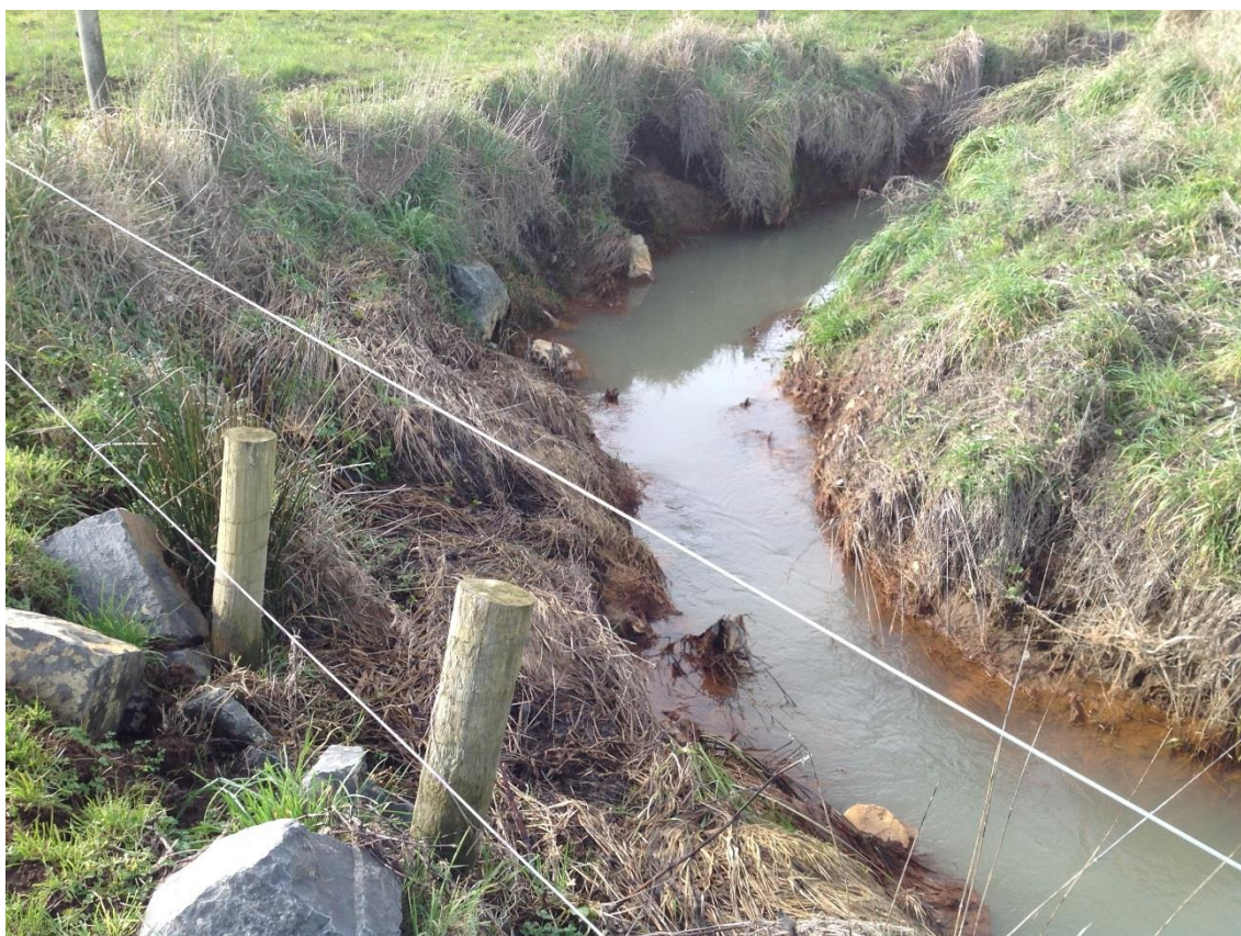
Plate 5: Rock armouring collapsing into the stream
