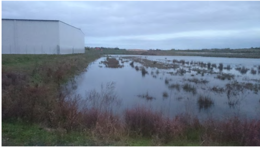
Figure 6-7: HJV Pond looking from the north
