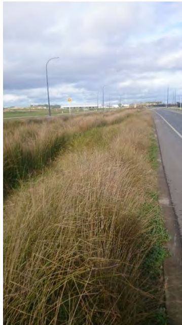
Figure 6-2: Central swale along the main road through the Porters development (looking south)
