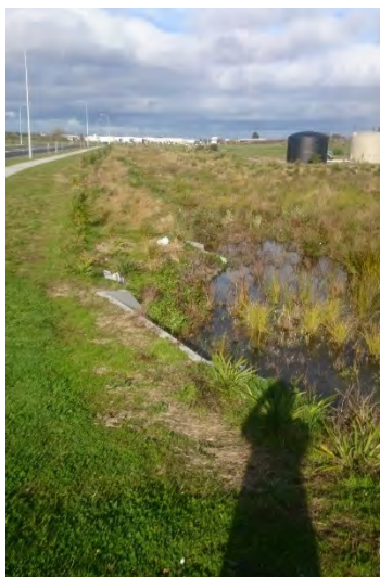
Figure 6-10: Swale C (along Arthur Porter Drive looking south)
