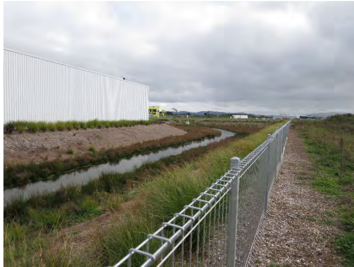
Figure 6-14: 4 Guys Pond (looking west)
