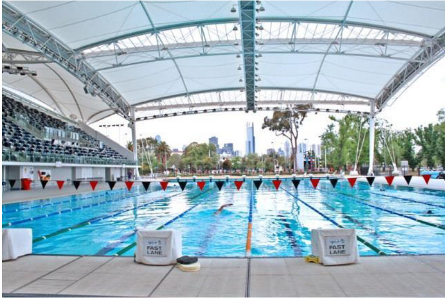
Figure 31: Hard top canopy over swimming pool
